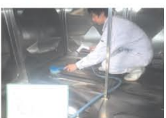
貯水(貯湯)槽清掃
